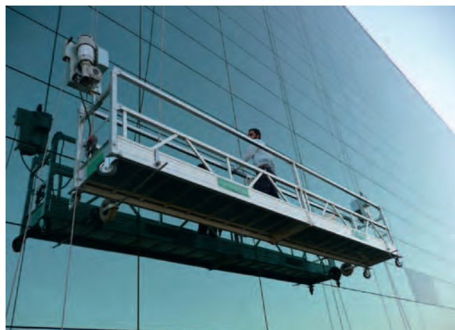
Figure 4. Plate-forme suspendue (© SFECE).
